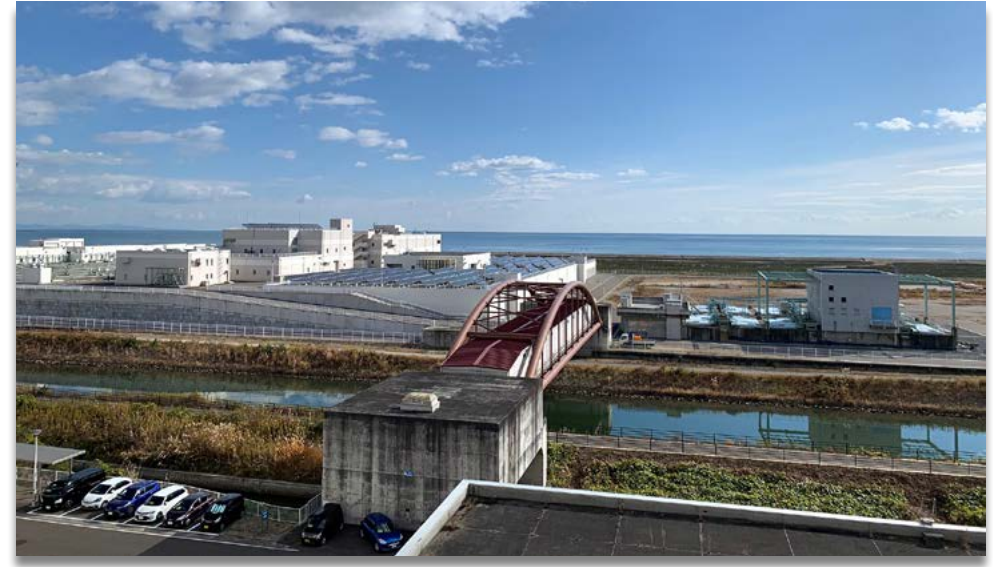
Figure 4: View on the Minami-Gamo Wastewater Treatment Plant after reconstruction
