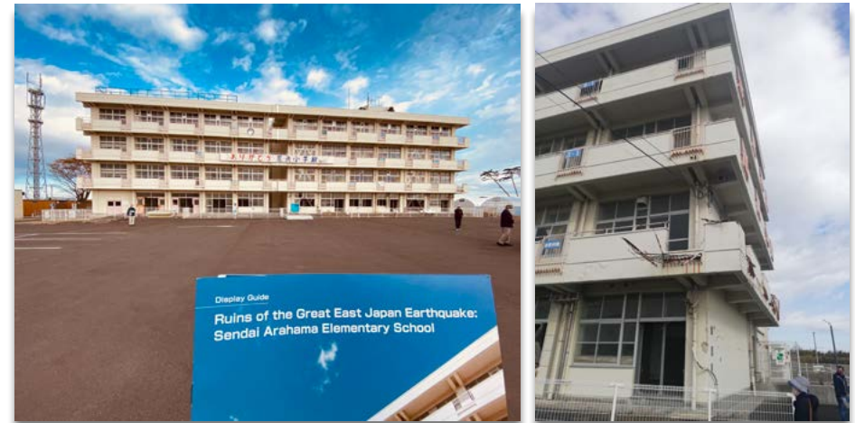
Figure 2: On the left side: Front view of the damaged Arahama Elementary School which saved 320 students and residents. On the right side: A close-up from the damages on the school.
