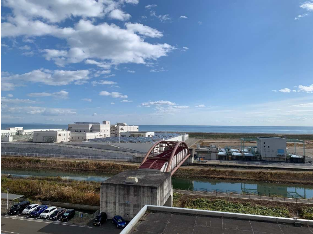
Figure 5: View on the Minami-Gamo Wastewater Treatment Plant after reconstruction
