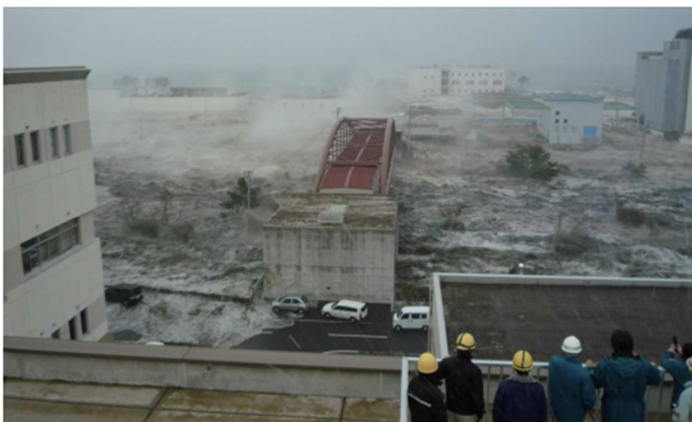
Figure 3: Flooding and evacuation of Minami-Gamo Wastewater Treatment Plant after the tsunami on March 11, 2011 (Sendai City Construction Bureau 2013).
